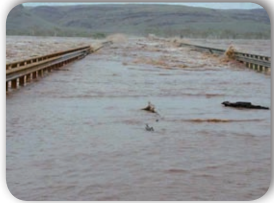
Using the control capabilities of Campbell loggers alarming conditions such as road signals can alert drivers of unsafe road conditions during flood events
